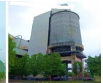
Dry fly ash unloading system
