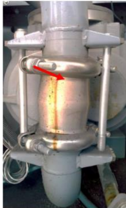
Leakages from joint set sealing area.
