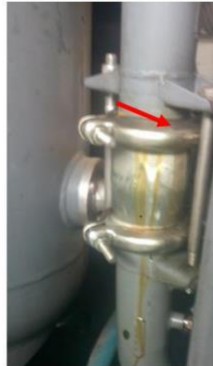
Leakages from joint set sealing area.
